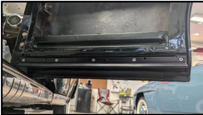
Door weatherstripping has been installed
